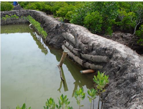
**Figure 2.** A pond at Majaoni showing stand pipe for draining the pond and overflow pipes to relieve the pond of extra water at spring high tides and increase water exchange in the culture ponds.
